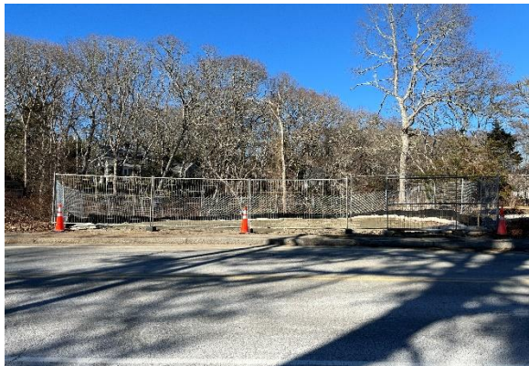
567 Shootflying Hill Road Pump Station
